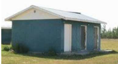
Washroom/ Shower Building
